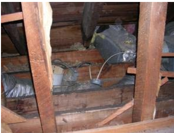
Low levels of insulation - note the exposed floor joist which is only a 2x4. Good insulation would be 12 inches or so.
