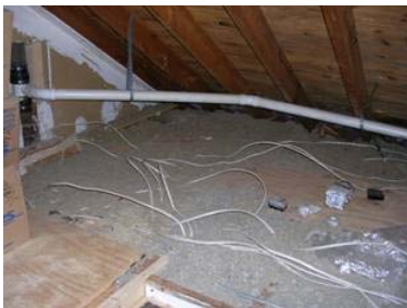
Low levels of insulation - note the exposed floor joist which is only a 2x4. Good insulation would be 12 inches or so.
