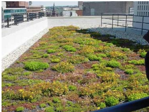
At Casey Trees Roof - 1425 K St NW
