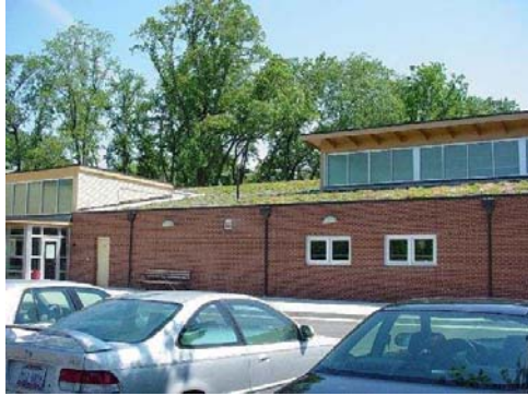
Walter Reed Community Center (Arlington)
