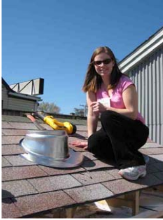
Green Building Institute Executive Director, Hannah Wood, helps install a Daylight Tube
